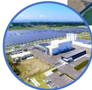
Energy Storage/ Hydrogen Production
