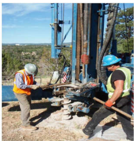
Groundwater monitoring wells will be installed under the Recovery Act
